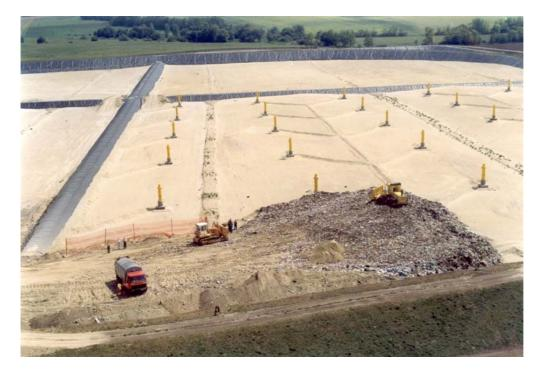
Figure 4: Aerial photo taken during the first placement of waste in 2000 with the gas wells
